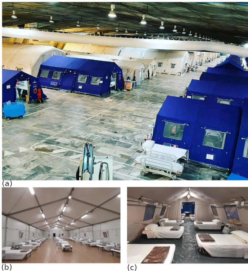
Figure 5.5 (a) Overview of the Valentino Field Hospital. (b)(c) Inside of the "rooms" built up with different types of tents.
