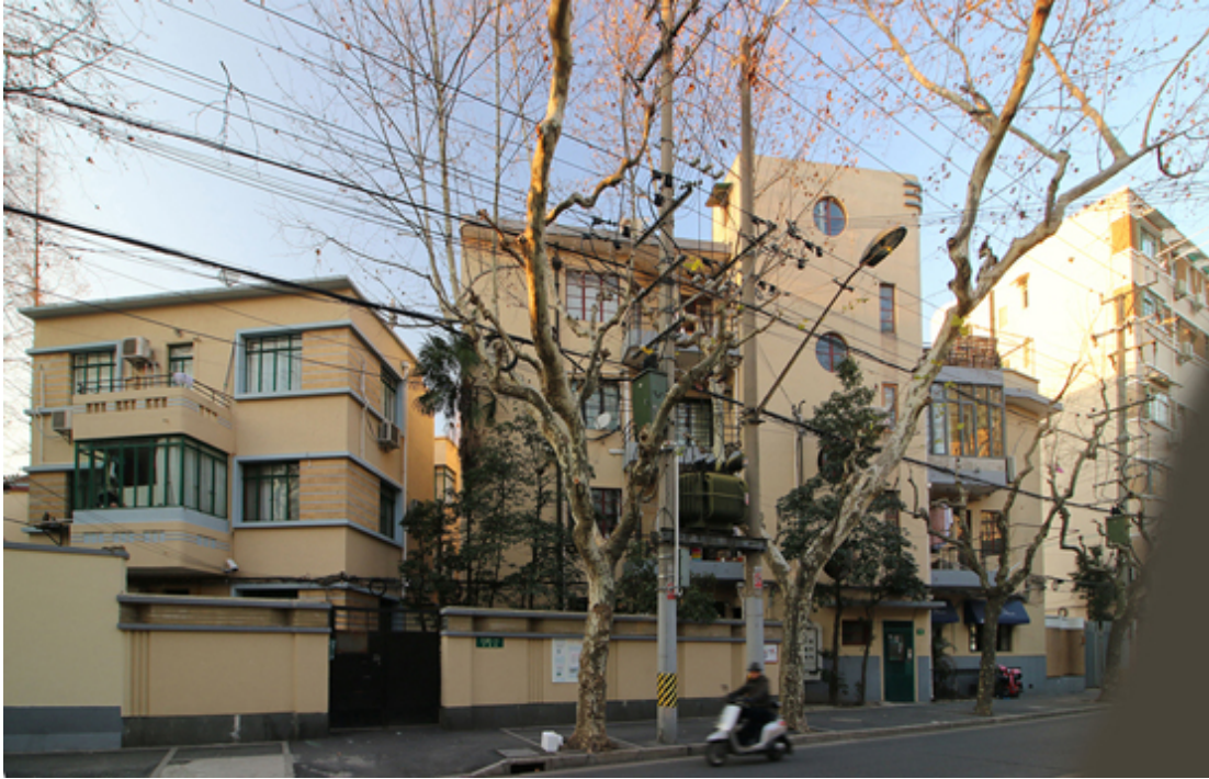
FIGURE 13.12: Katya Knyazeva, Art Deco apartment buildings on Yongfu Road , designed by (left to right) I. Tomashevsky, V. Kooklin and N. Emanoff respectively, Shanghai, 2018.
