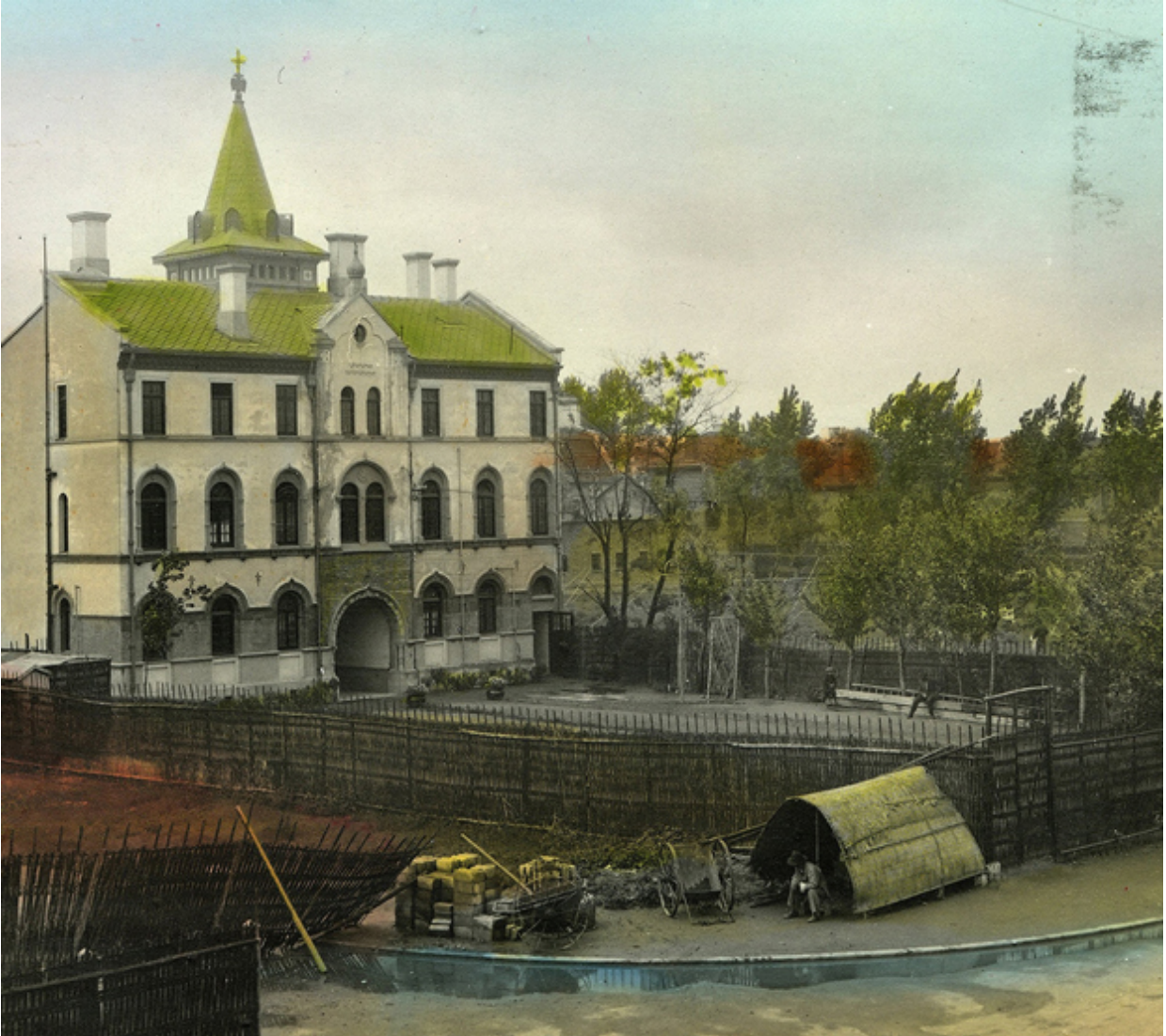
FIGURE 13.10: Bishop Apartments , designed by Alexander Yaron, and the site prepared for the construction of the Orthodox Cathedral, Shanghai, c.1933, Russian Spiritual Mission in Beijing.
