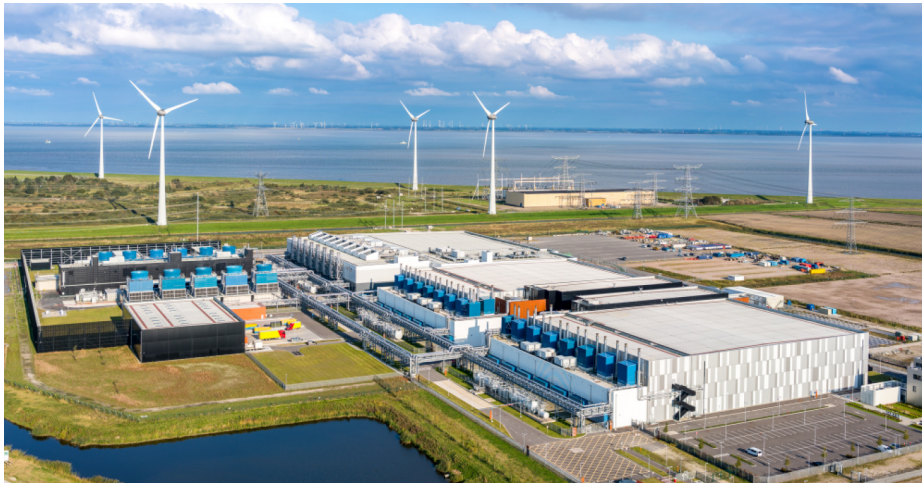
Figure 2.2: Google's data center campus in Eemshaven, Netherlands
